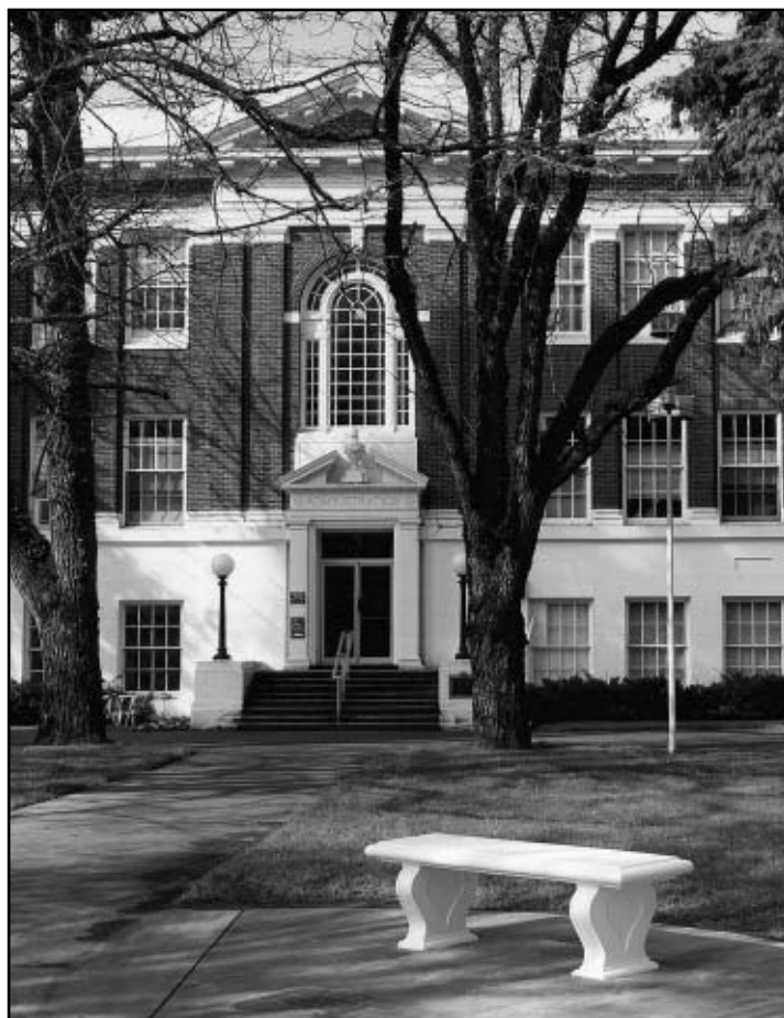
Figure 1. The Albany Research Center main building.
